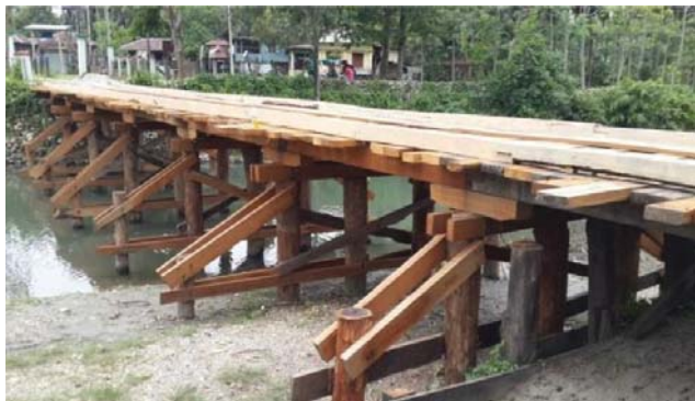
Construction of wooden Bridge-Hollong
