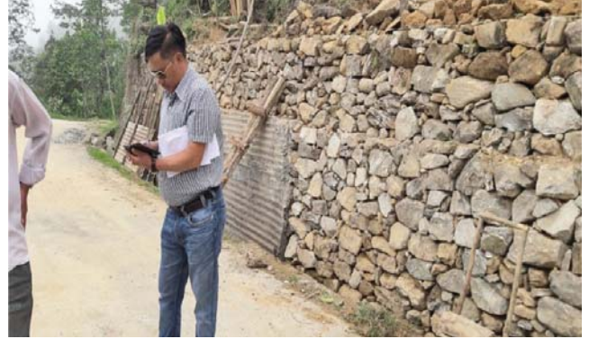
Protection Wall Rampuria
